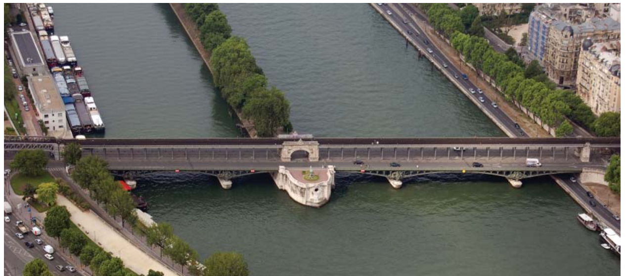
An elevated Paris metro line crosses the Seine, sharing a bridge with street traffic.
